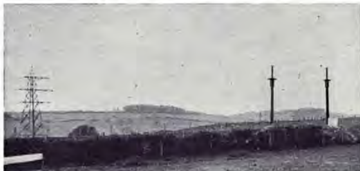
A variation of the 'Trident' line technique in use here to lift some 132 kV tower lines clear of a road at Llandegai, near Bangor.
